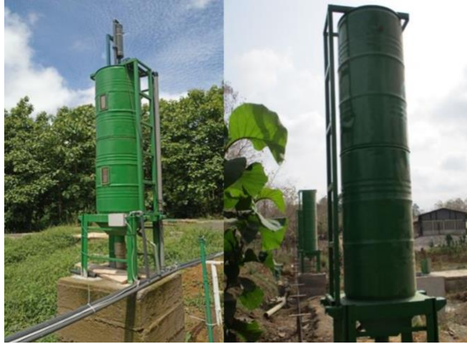
Device for storing filtered biogas in biogas tanks, produced locally by SEFT-AFRICA
